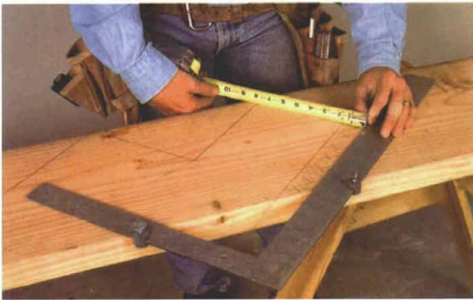
Subtract the thickness of a tread. For the bottom rise to be the correct height, the thickness of one tread must be subtracted from the bottom of the stringer. Moving the square to the other side of the stringer makes it easier to complete the lines.
